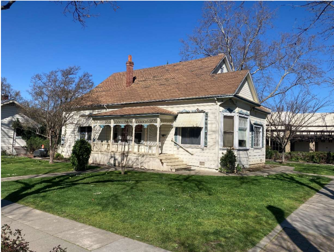
Figure 3 – 305 E Street, view facing northwest (ESA 03/07/2024)
